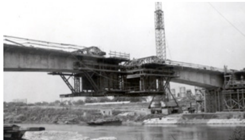
The Moson Danube Bridge at Győr, the first cast in situ balanced cantilever bridge in Hungary, 1978
