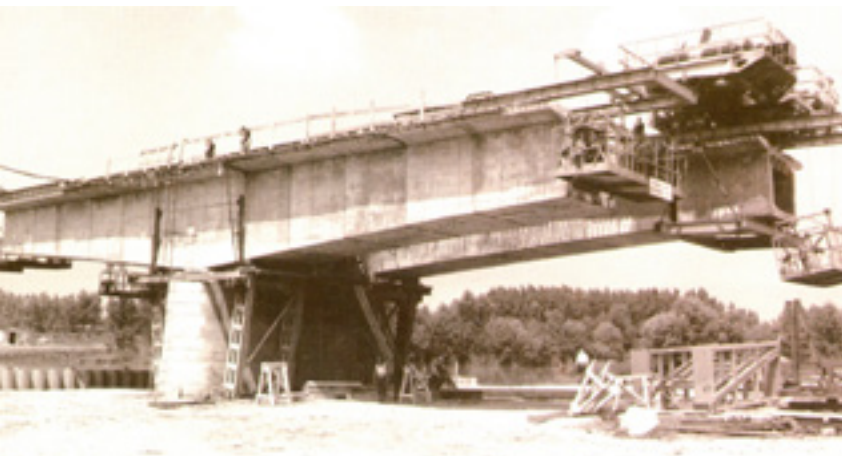
Kunszentmárton, our first prefabricated segmental balanced cantilever prestressed reinforced concrete bridge, 1975
